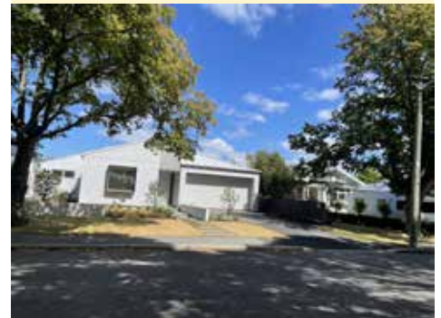
Fitting in or sticking out? Modern building adjacent to an American style bungalow. Residents in the heritage area fear modern developments like this could erode the area's special character and lead to removal of protection homes in the area enjoy
