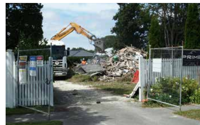
This Geraldine St Villa is being replaced by several modern units
