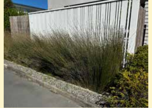
A swale in Packe St
