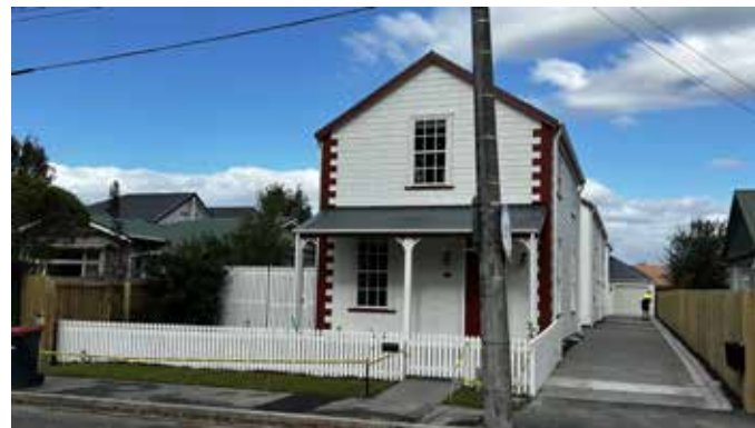
New Brookfield build on Edward Avenue
