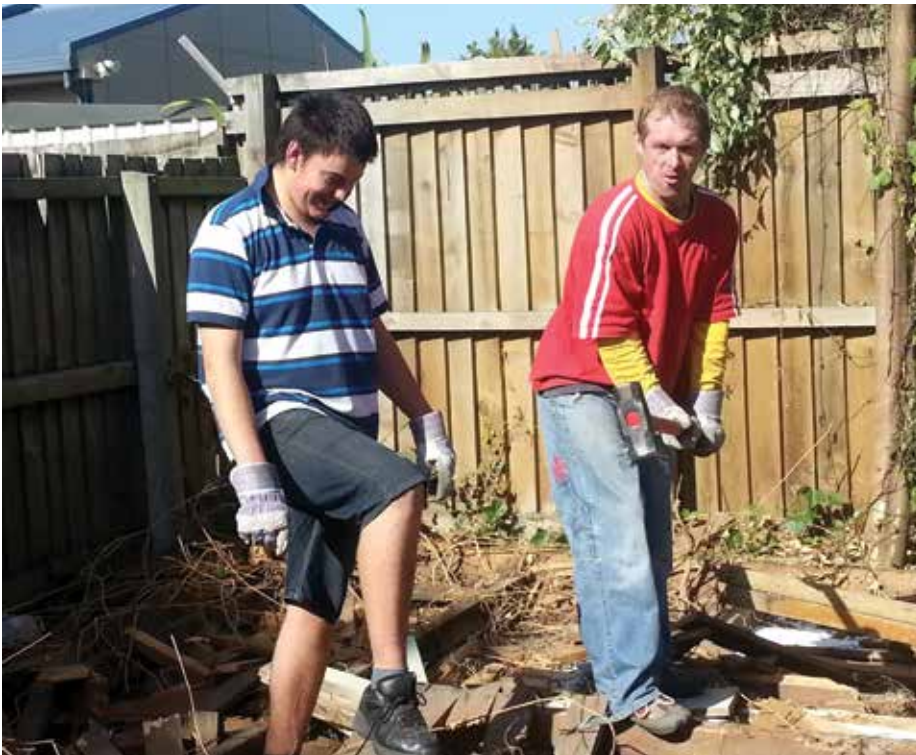
Ben and Liam with the remains of the shed at 130 Caledonian Road after they dealt to it with a sledgehammer.
